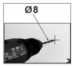
**3)** Using a drill bit with a 8 mm diameter, make holes in the wall on the positions that you have marked in step 2.
