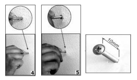
4) Insert rawl plugs into all of the holes that you have drilled.
