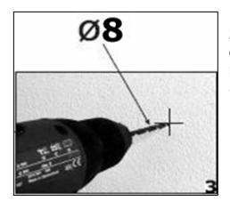
**3)** Using a drill bit with an 8 mm diameter, make holes in the wall on the positions that you have marked in step 2.
